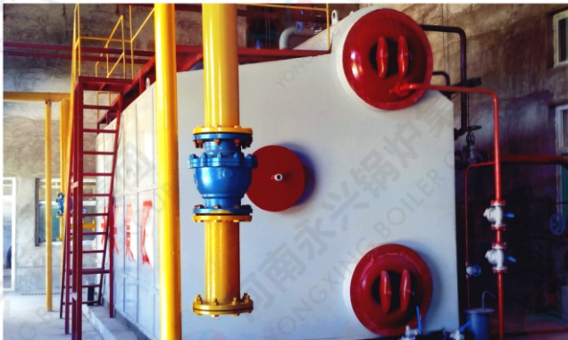
2018.04.10 山西喜跃发集团6吨燃气过热蒸汽锅炉 2018.04.10 6t/h super steam boiler in Shanxi Xiyuefa group
