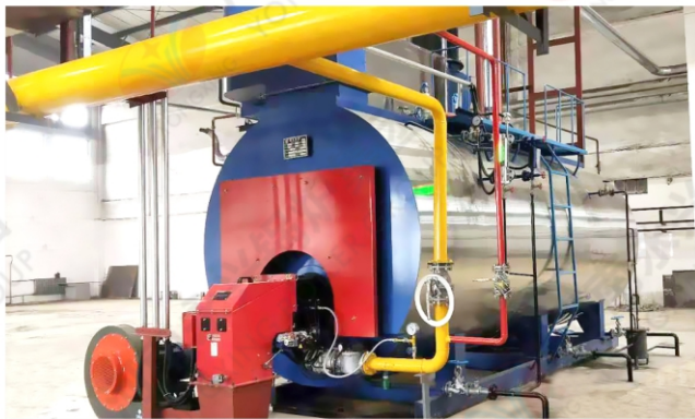
2018.09.21 神华集团6台10吨冷凝蒸汽锅炉 2018.09.21 6 sets of 10t/h condensing steam boilers in Shenhua group
